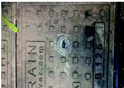
Condition of the socket type keyhole lifting arrangement of THERMODRAIN FRP manhole covers
